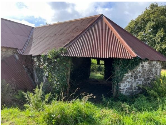
F - Roundhouse attached to original structure
