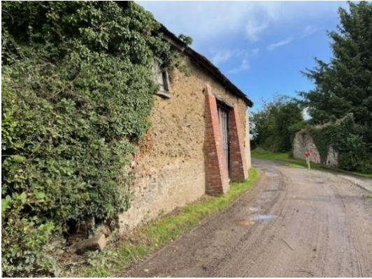
C - Threshing barn built of cob
