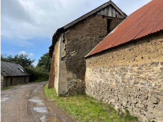
D - Later addition to threshing barn built with stone and cob
